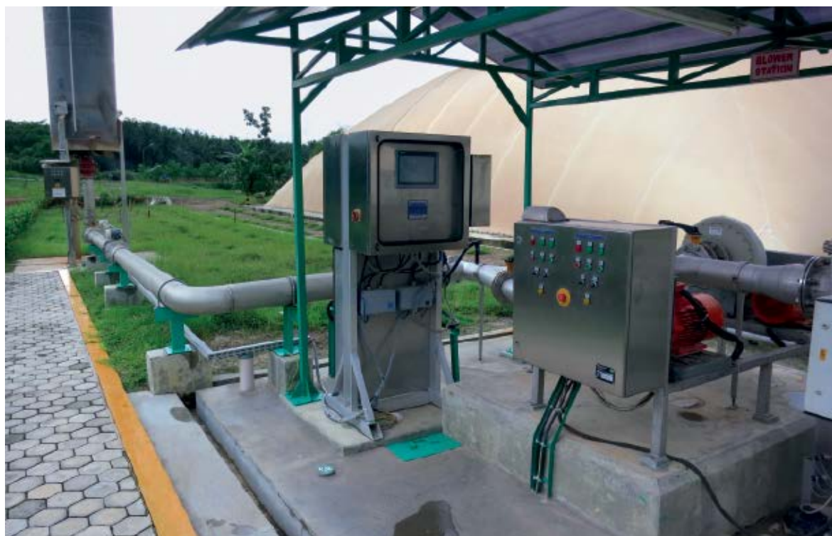
The INCA gas analysis system measures the composition of natural gas – here in a biogas plant in Indonesia. (Photo: Torsten Haug)
