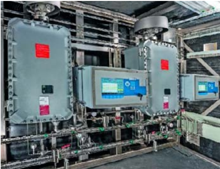
The CWD2000 Ex as a dual instrument enabling redundant measurements
